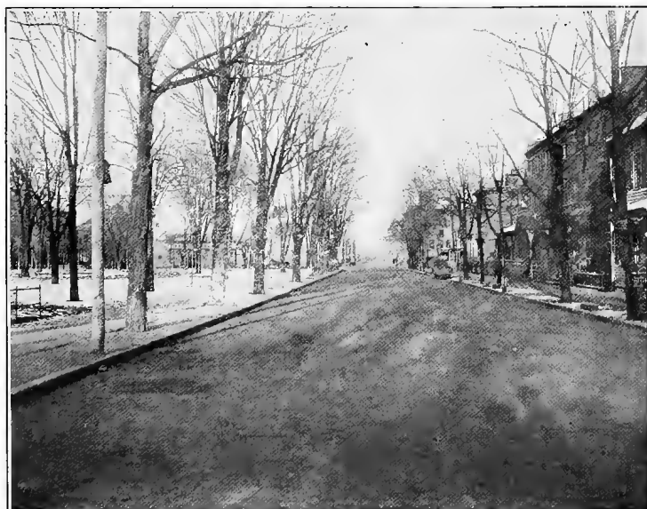
MAPLE STREET, HOLYOKE, MASS., 1901. Before and after paving with Bituminous Macadam.
